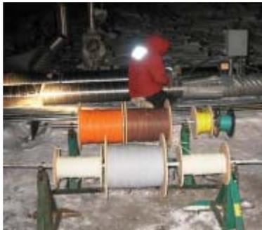
Figure 2 Electrician pulling new heat trace and control wires for McMurdo water lines.
