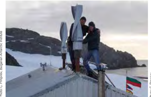
Installing wind generators on roof of main station building
