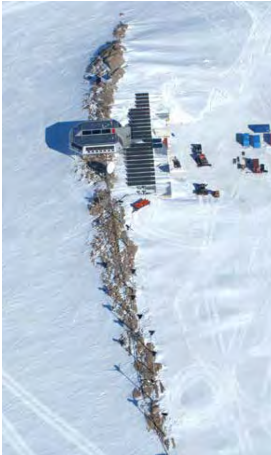
Princess Elisabeth Station and wind turbines
