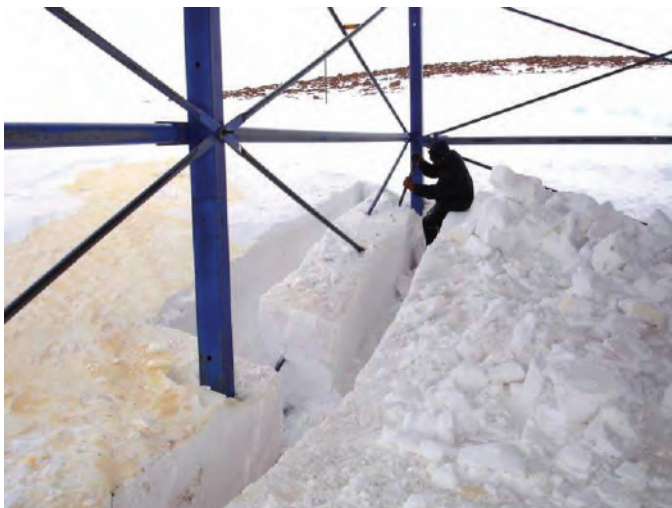
Figure 2: trenches being dug in the contaminated area of the spill
