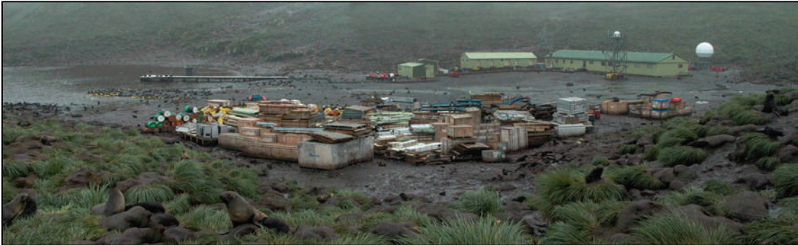
Figure 7: Removal of waste cargo at Bird Island
