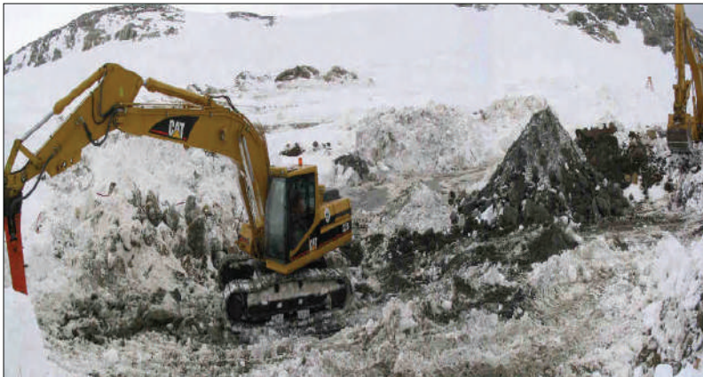
Figure 6: Excavation of frozen waste from Thala Valley
