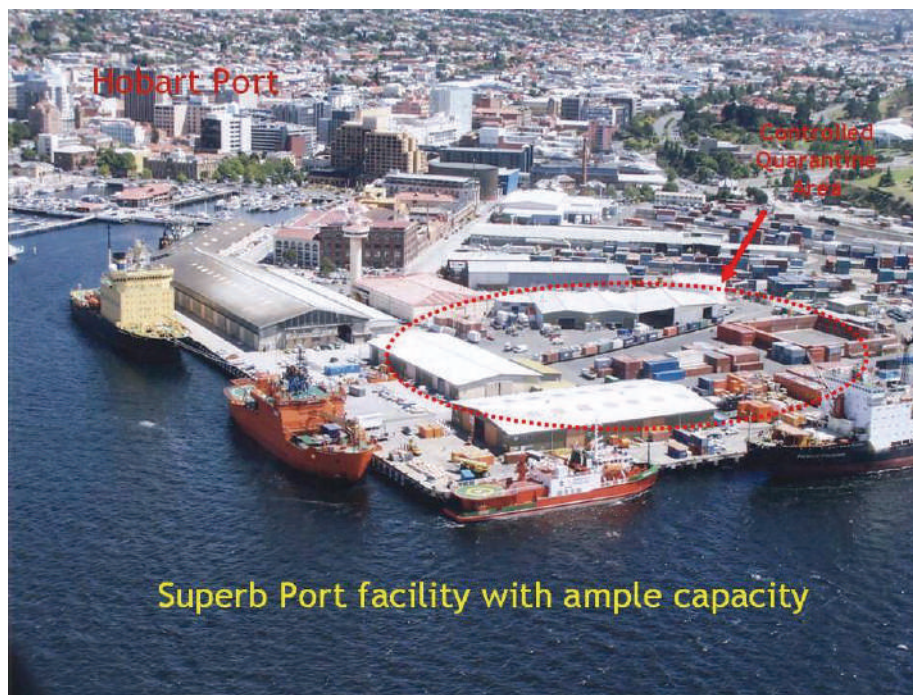
Figure 1: Superb port facilities used by Veolia / Collex in Hobart
