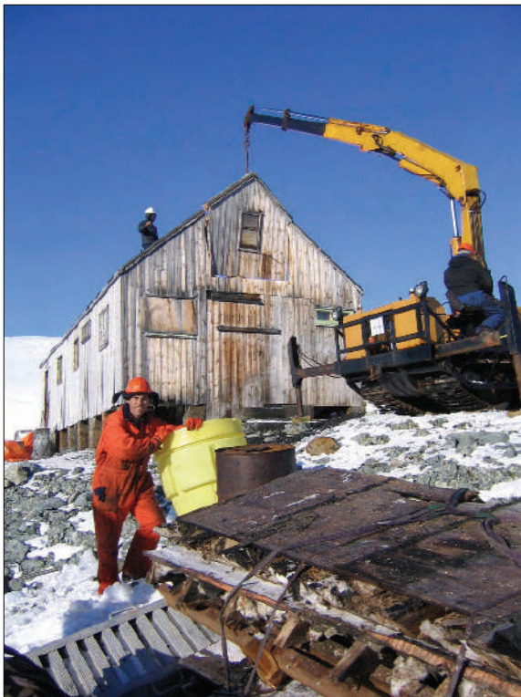
Figure 6: Demolition starts at Prospect Point.
